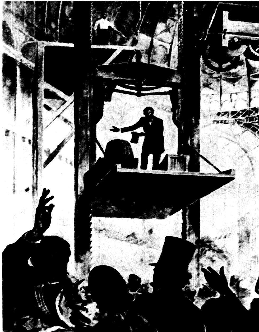
OTIS DEMONSTRATED ELEVATOR'S SAFETY AT CRYSTAL PALACE BY CUTTING ROPES
