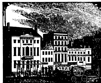
Tammany Hall, left, and building farther up Nassau St. were later homes of paper.
