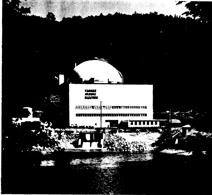
New atomic-powered generating station in Mass. Westinghouse Electric designed and developed the reactor.
